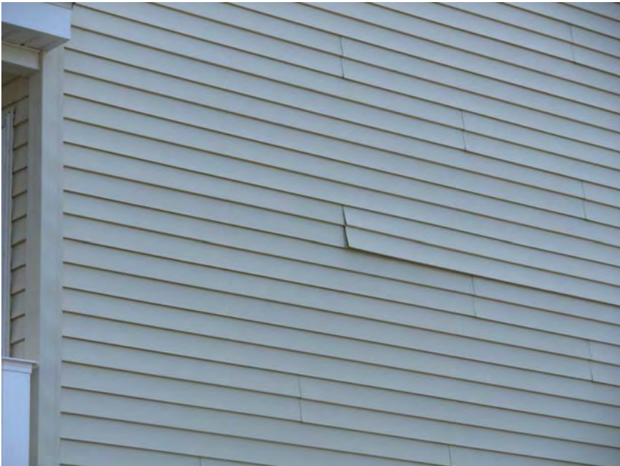
3. Spot vinyl siding damage
