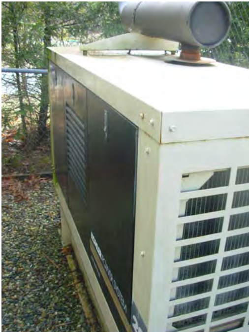
11. View of the generator serving the sewage ejection pumps
