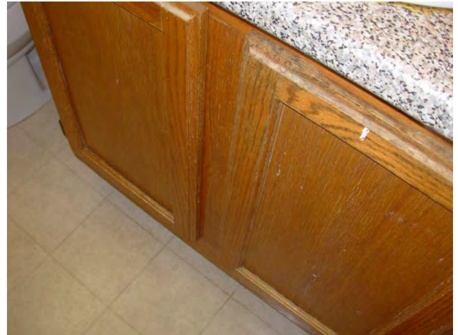
16. Typical finish wear at older vanities and kitchen cabinets
