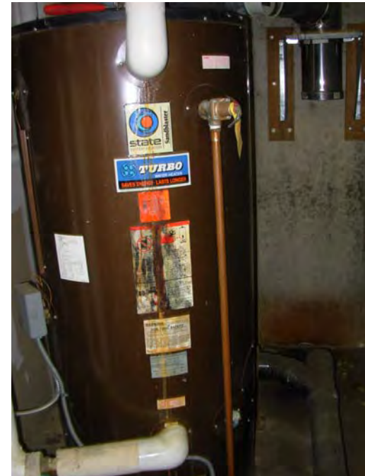
12. DHW tank serving the laundry facility
